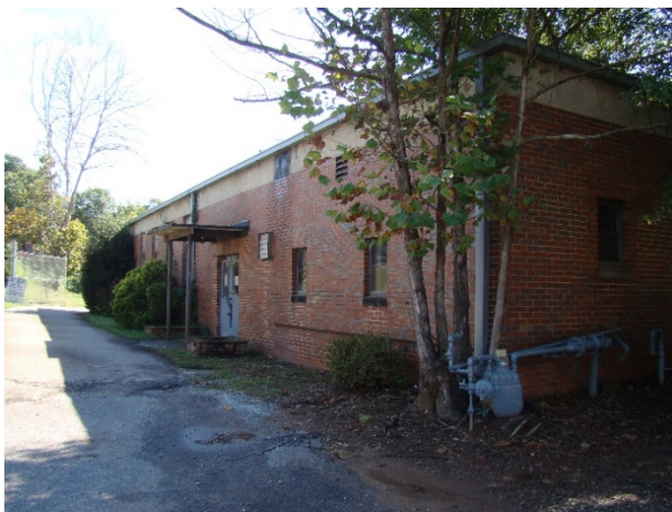
West Broad façade/entry
