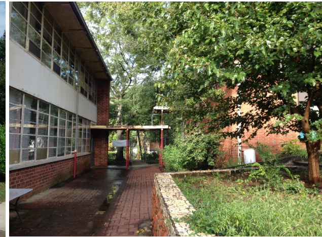
Plaza façade @ canopy/building connection
