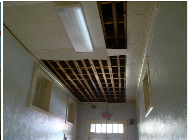
Wood roof framing above ceiling
