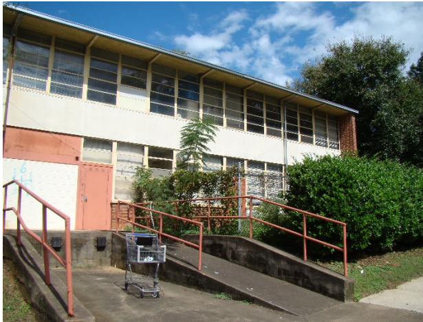
Campbell Lane façade/loading
