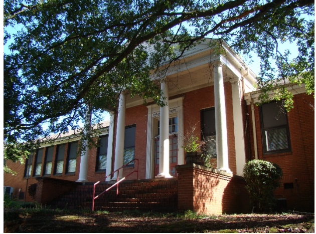
Minor Street façade/entry
